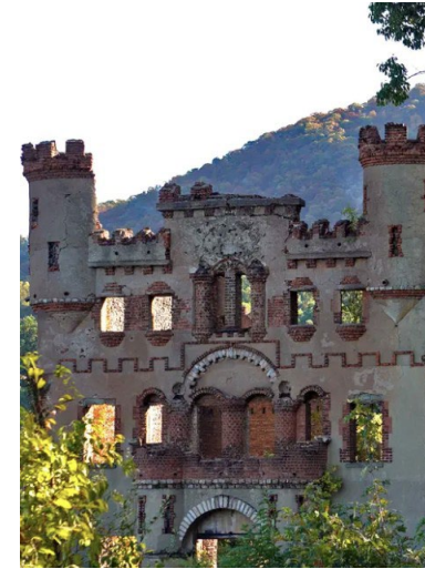
11 The warehouse wall
