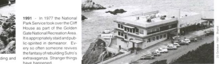
1991 - In 1977 the National Park Service took over the Cliff House as part of the Golden Gate National Recreation Area. It is appropriately staid and public-spirited in demeanor. Every so often someone revives the fantasy of rebuilding Sutro's extravaganza. Stranger things have happened.
