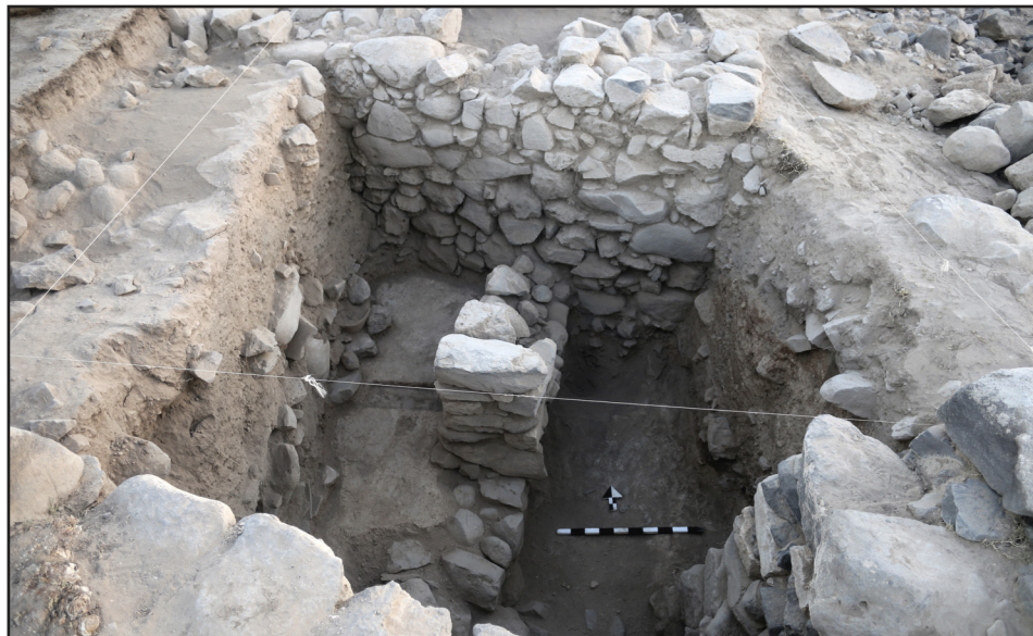
Wall Between Rooms and Plasterd Surface (1).
