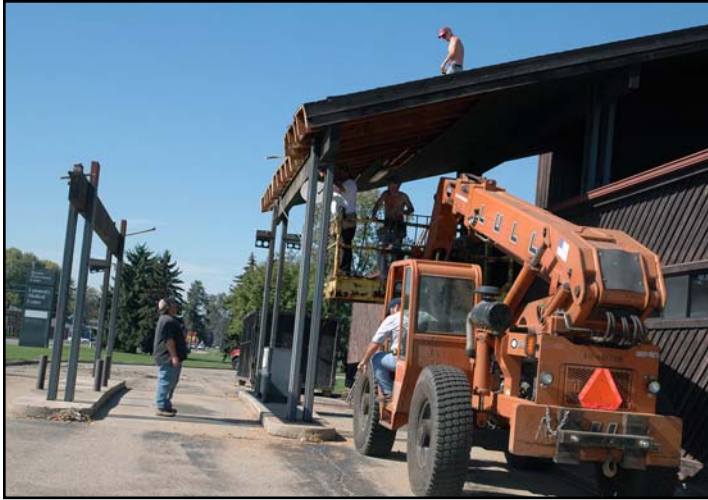
Workmen Remove Awning from Front of the Museum.
