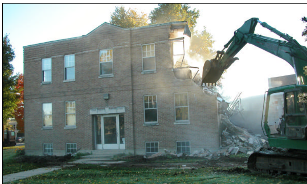
Demolition of the old Institute of Archaeology/Horn Archaeological Museum.
