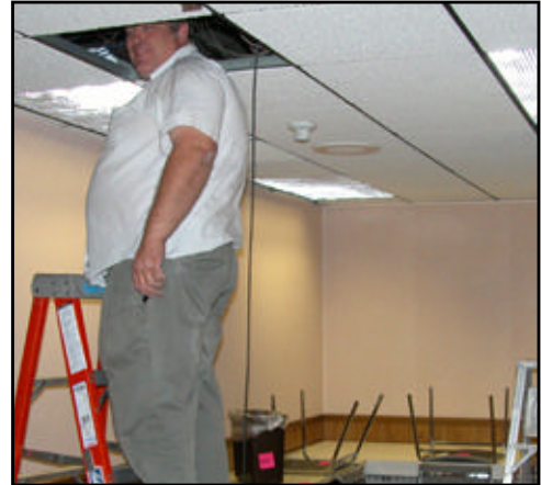
Reginald Swensen installs new internet lines.
