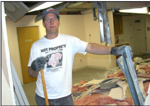
Brooks Payne demolishes area for the new classroom.
