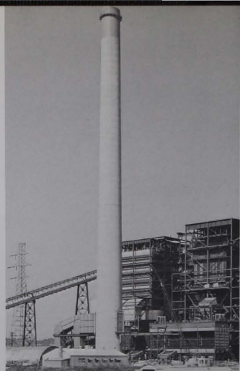
Penna. Power & Light Co. plant
