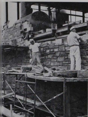
Stone masons working on the west side of the power plant.
