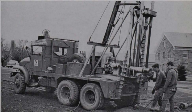
Preliminary borings at the site of the new power plant
