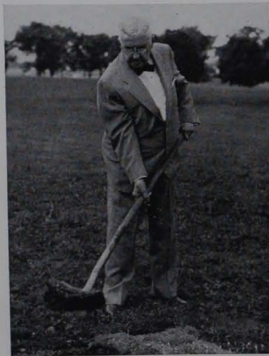
Dr. Paisley, breaking ground in June, 1955, for the women's dormitories. He is shown here using the shovel which was used to break ground for Bomberger Hall in 1891.
