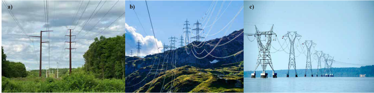
FIGURE 3.3 Difficult operating areas such, a) shrubs below the lines[43], b) mountainous terrain [3] and c) power-lines river crossing [15].
