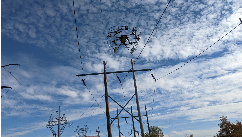
FIGURE 3.19 NADILE with a set of un-energized power lines mock-up.
