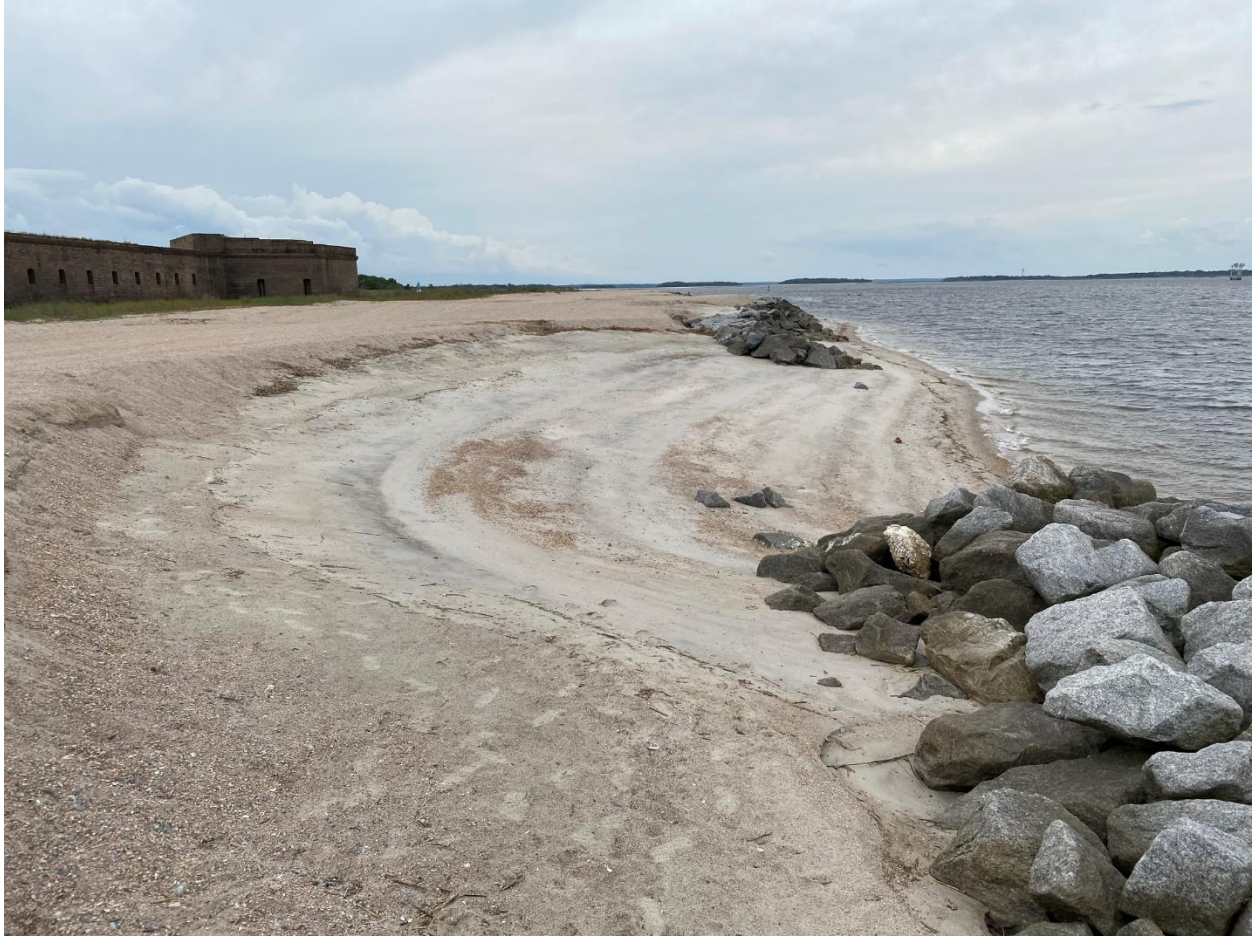
Figure 22: Erosion between rock groins on the shoreline near Fort Clinch. (Author's photo)
