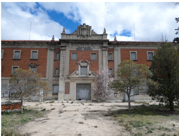
Fig. 5. General Monasterio barracks before the redevelopment works of summer 2022.
