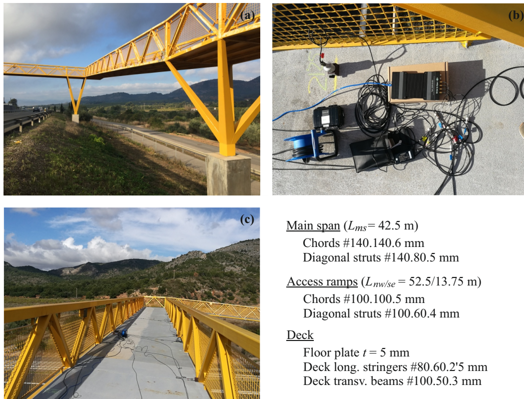
Figure 2. Footbridge under study.
