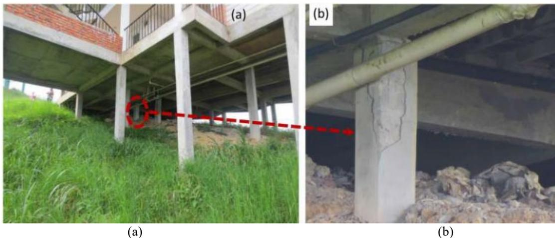
**Fig. 4 - A three-storey RC building on sloping ground (a) short column phenomenon with short and long columns, and; (b) shear crack damage at shortest column**
