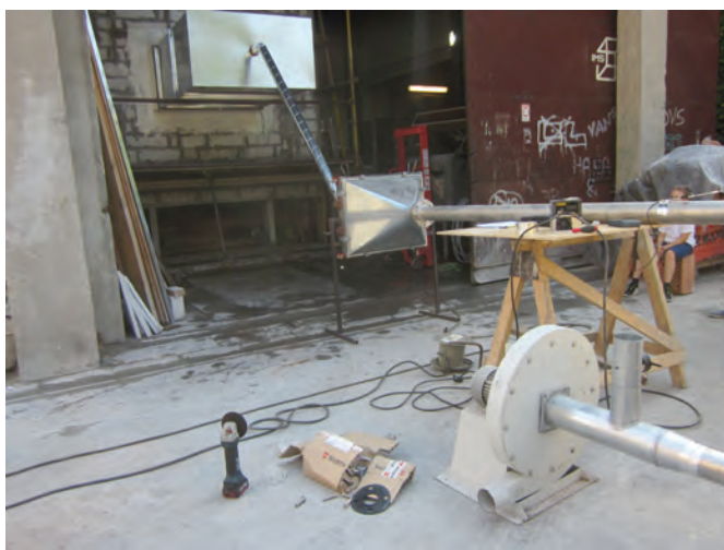
Figure 6: Test equipment installed in Laboratory
