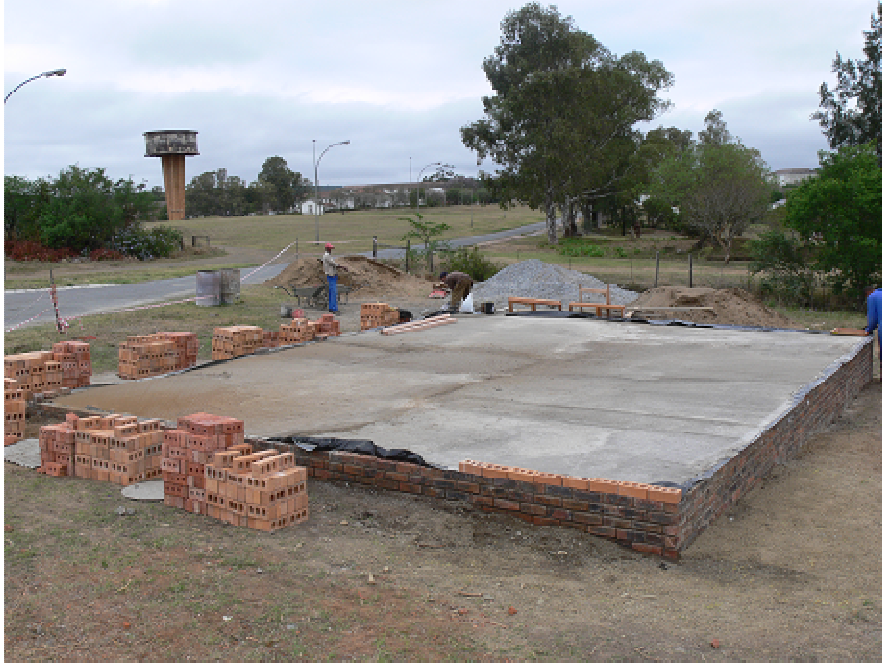
Figure B.4 The completed slab.
