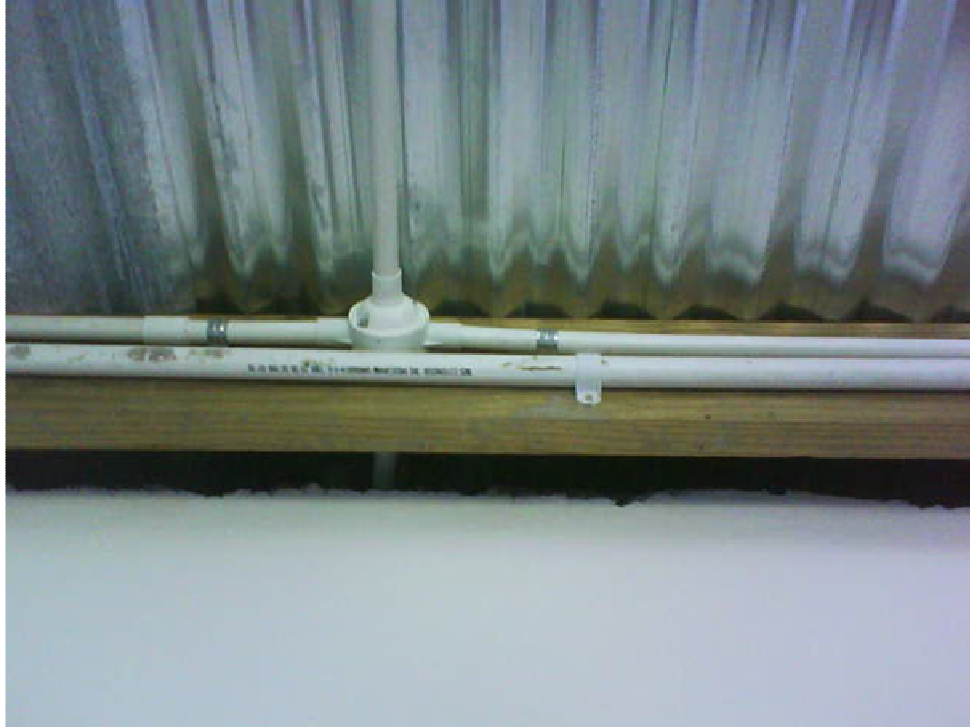
Figure B.8 Corrugated metal sheets, roof truss and electrical conduit
