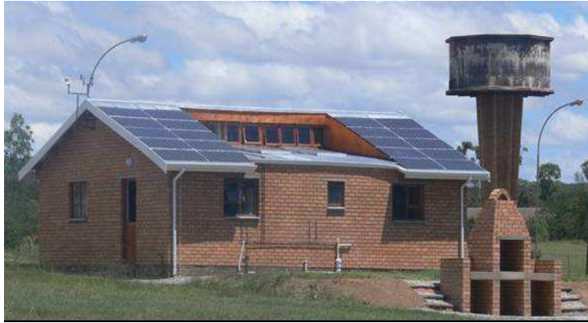
Figure 4. 6 The completed EEBIPV house (March 2009)
