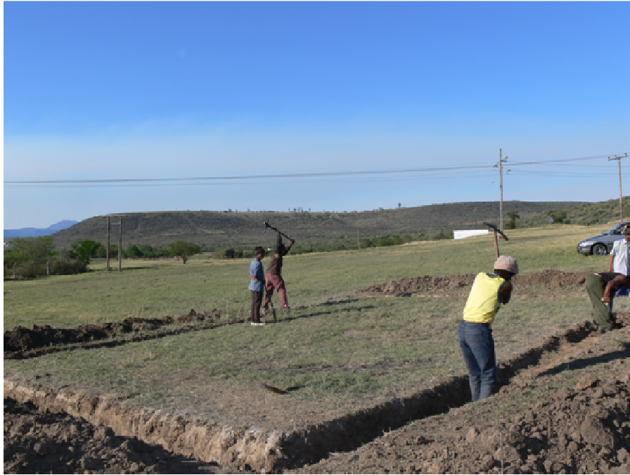
Figure B.2 Foundation excavation on first day.
