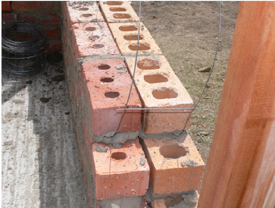
Figure B.6 The outer wall and steel reinforcement
