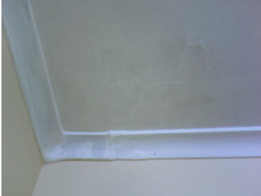
Figure B.12 The completed ceiling
