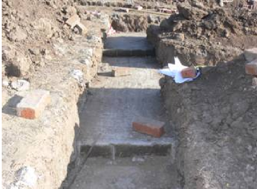
Figure B.3 The step footing.
