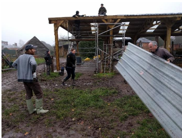
Figure 10-1: Helping with the barn roof at Canon Frome Court cohousing
