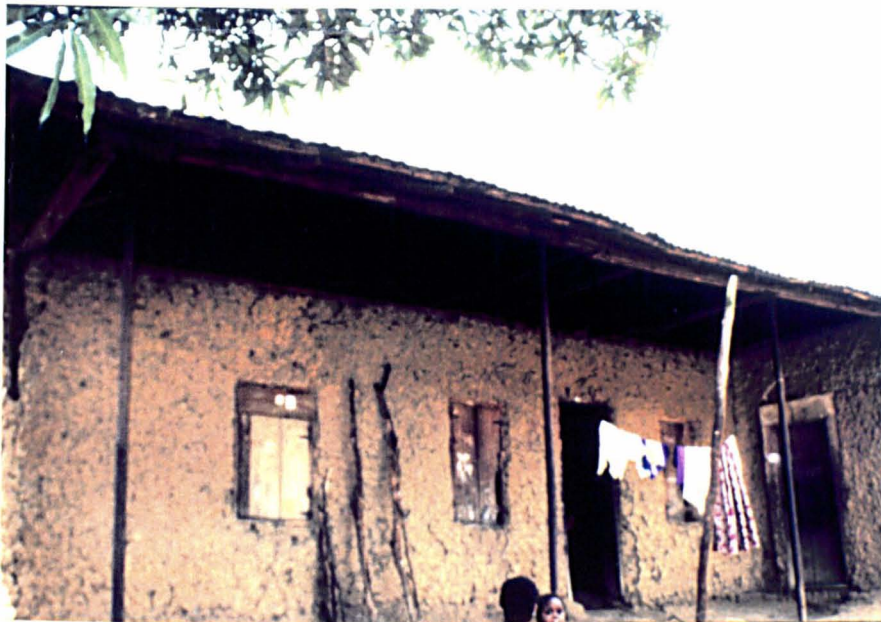
A: Mud and stick house with open eaves and no ceiling.
