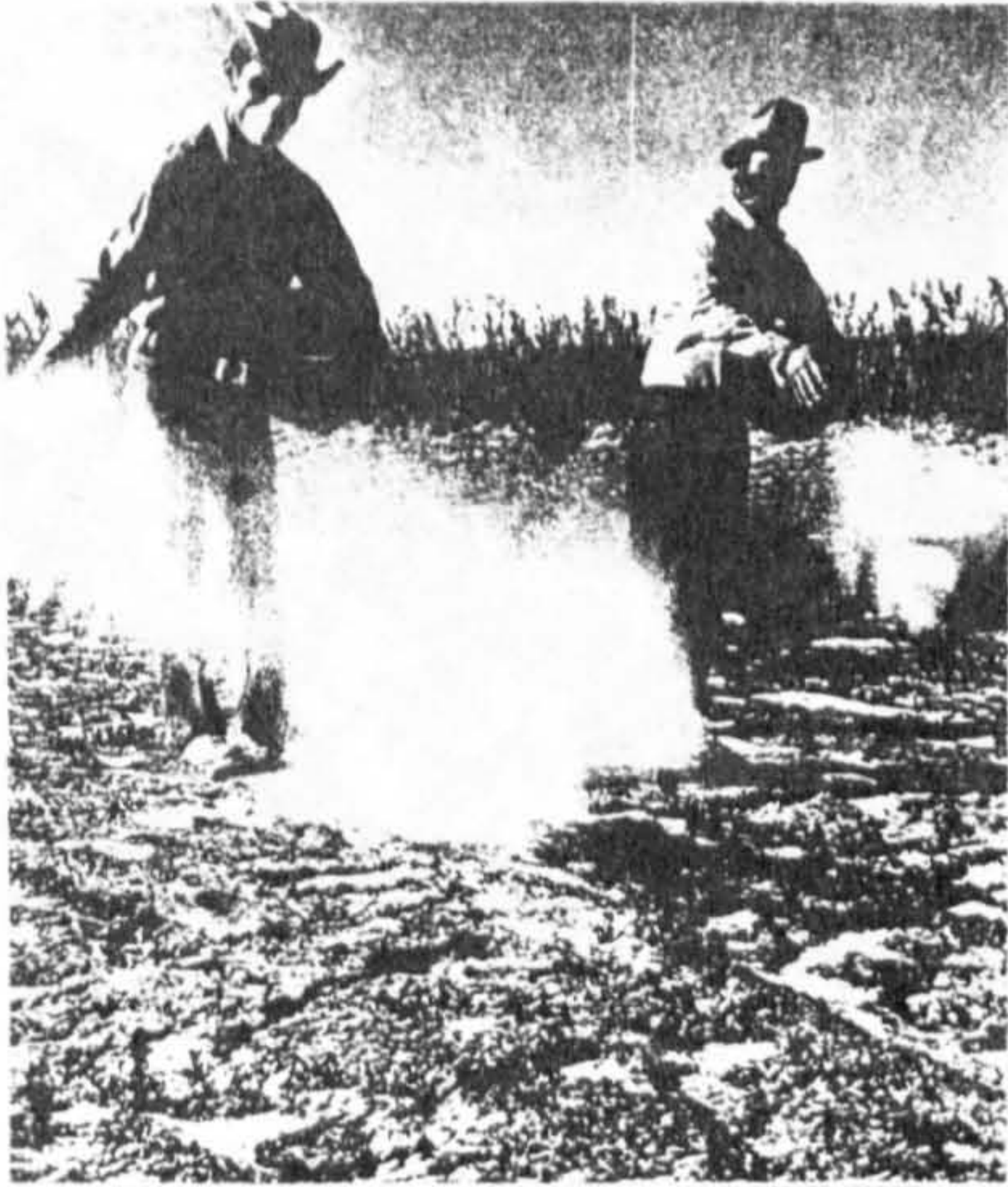
Fig. (8) Cracked soil structure indicates high calcium content in a dry pond bed in Coconino National Forest, Arizona. Water seeps away through the cracks. Rocks & weeds were cleared, and 1 ton of sodium carbonate applied by hand to 1000m 2 . This was mixed with the soil to a depth of about 8cm with a small tractor which caused the clay aggregate to break down into fine particles which sealed the pond bed (U.S. Dept. of Agriculture).
