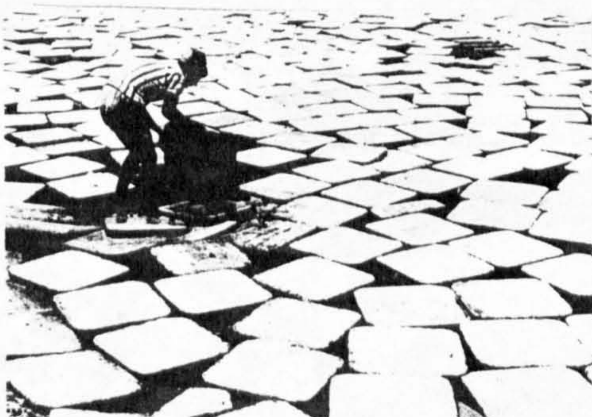
Fig. (7) Protective covering of lightweight slabs of polystyrene, sand and concrete, cut evaporation by about 80%. Exposed surface of each slab is painted white to reflect the intense sun rays. Submerged portion is coated with bitumen for durability and to avoid affecting the taste of the water. (National Institute for Water Research, South Africa).
