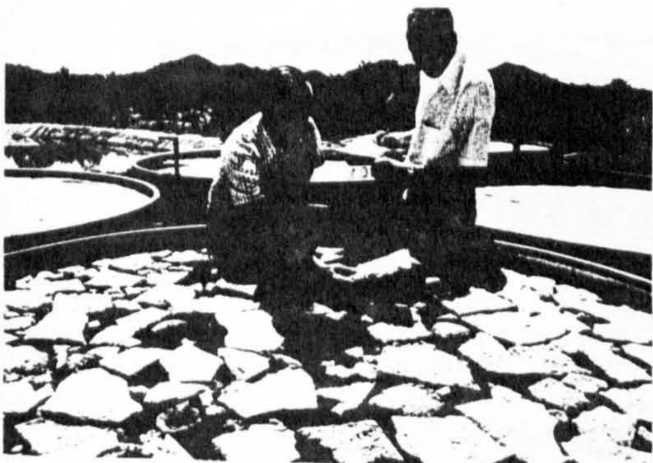
Fig. (6) Paraffin wax is shredded and spread for rainwater harvesting in Arizona. Melted by the sun, the wax flows into and seals soil pores (U.S. Dept. of Agriculture).
