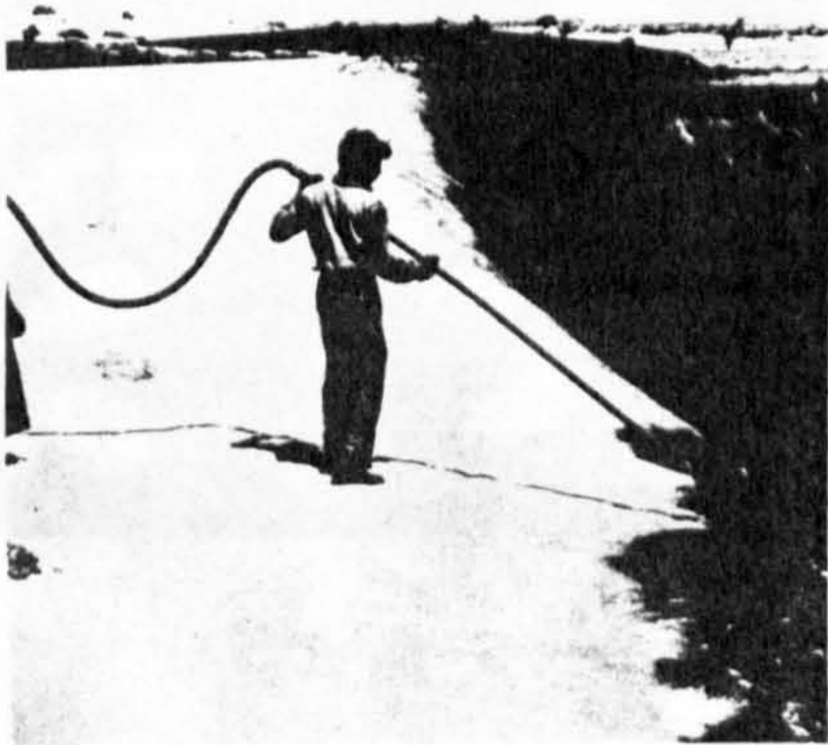
Fig. (10) Stabilizing dunes with a heavy oil mulch in the Rajasthan Desert, India. Unstabilized sand would either bury the young plants or blow away, exposing their roots (Exxon).
