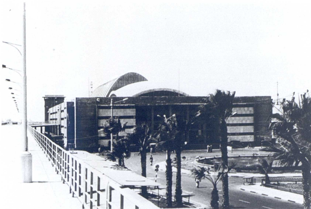
Figure 5.9: The building of maritime passenger station. It is considered to be the main complex of offices and services activities which is urban activity, as well as some commercial activities (antiques shops). It has also some administrative offices for port management and shipping lines which are public administration.
