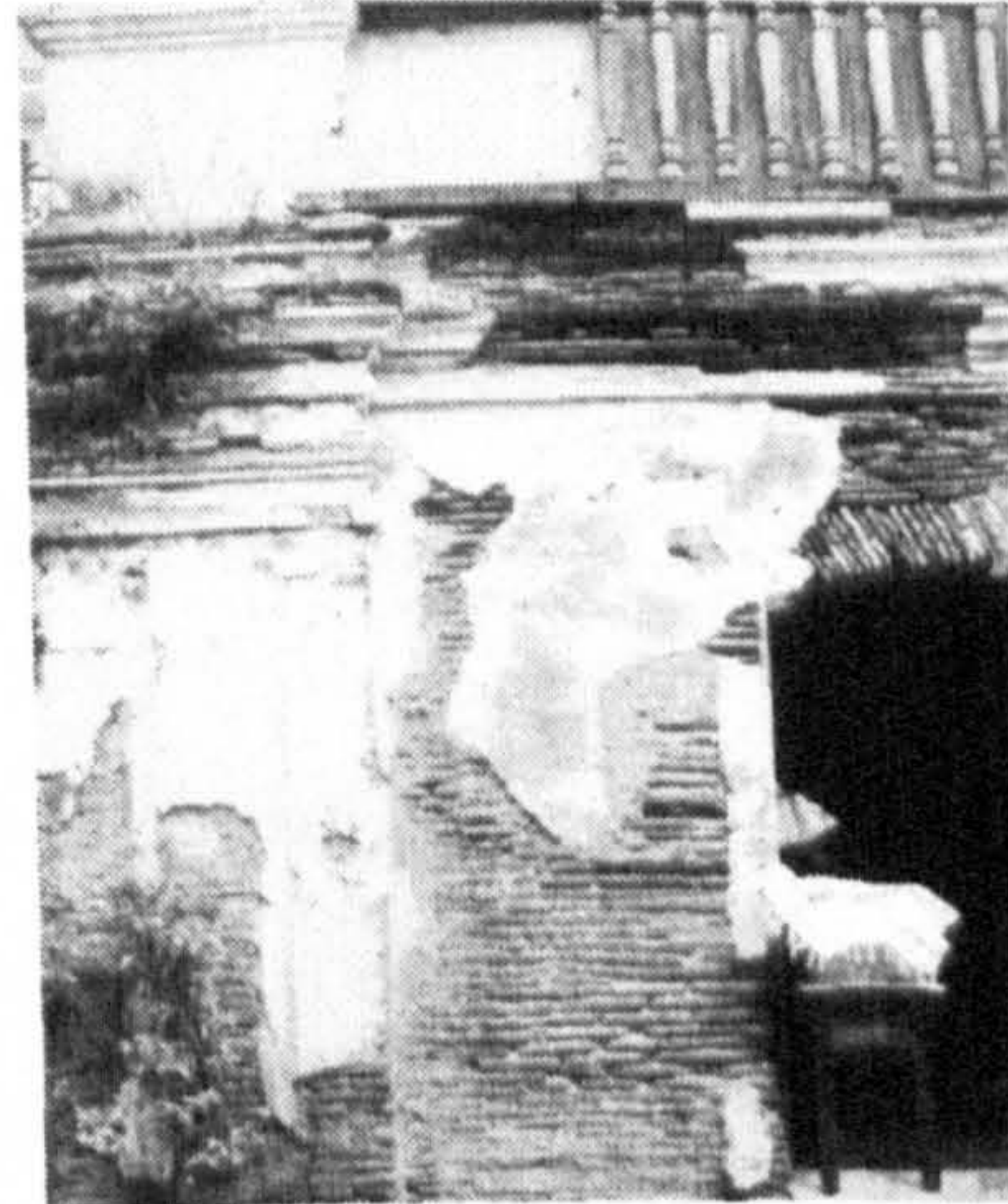
Exposed brick works
