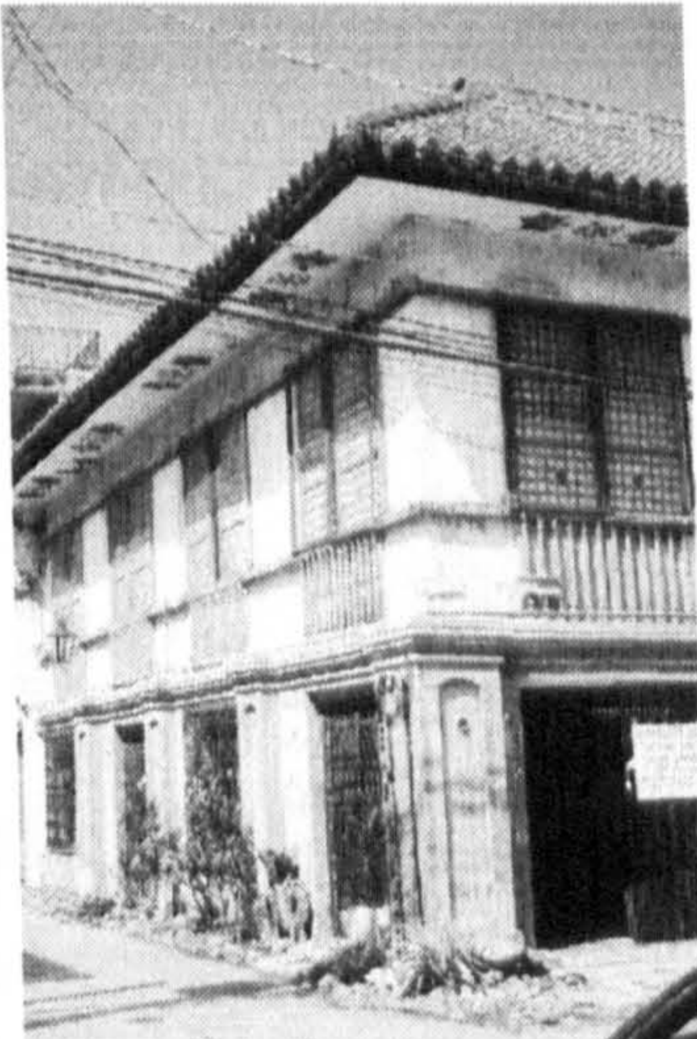
Figure 6.12: Straight façade with the walls on the upper floor flush with the ground floor.
