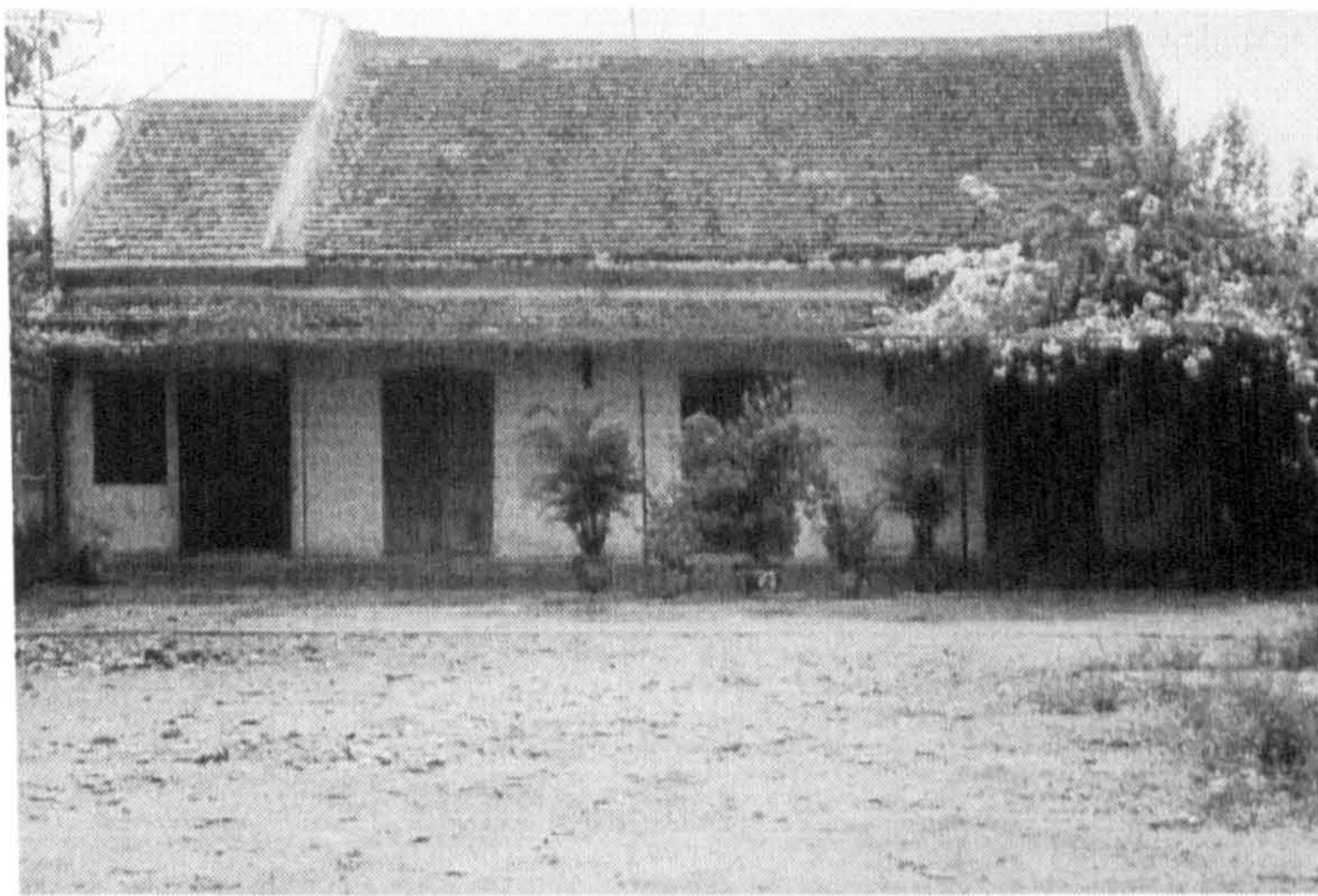
Figure 5.2: Main office of the Centre for Monument Management and Preservation on Le Loi Street.
