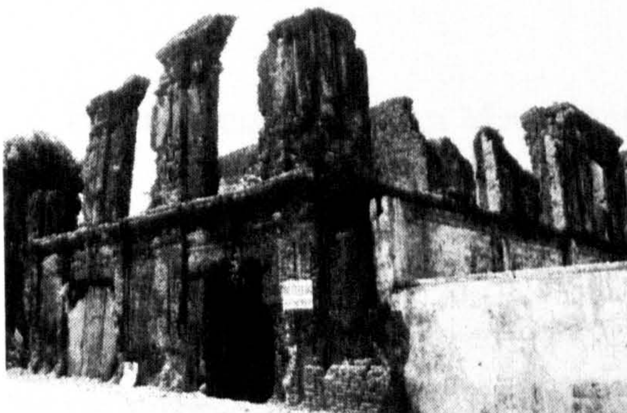
Figure 8.4: A ruined ancestral house on De Los Reyes Street. To one extreme, there are several houses are left in ruined. (Source: VMPlan, 2001)
