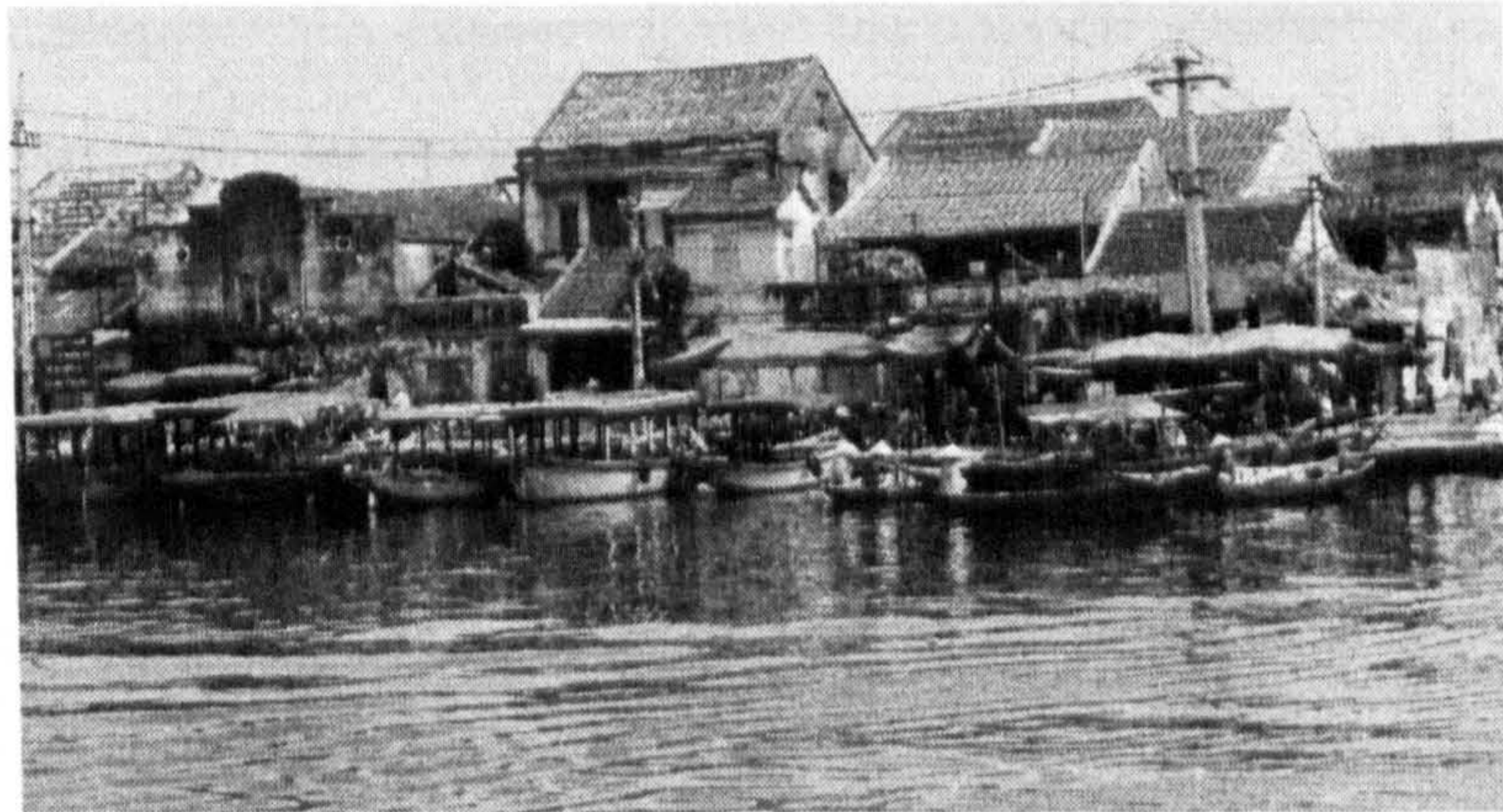
Figure 1.6: Two storeys shophouses dominate Hoi An waterfront
