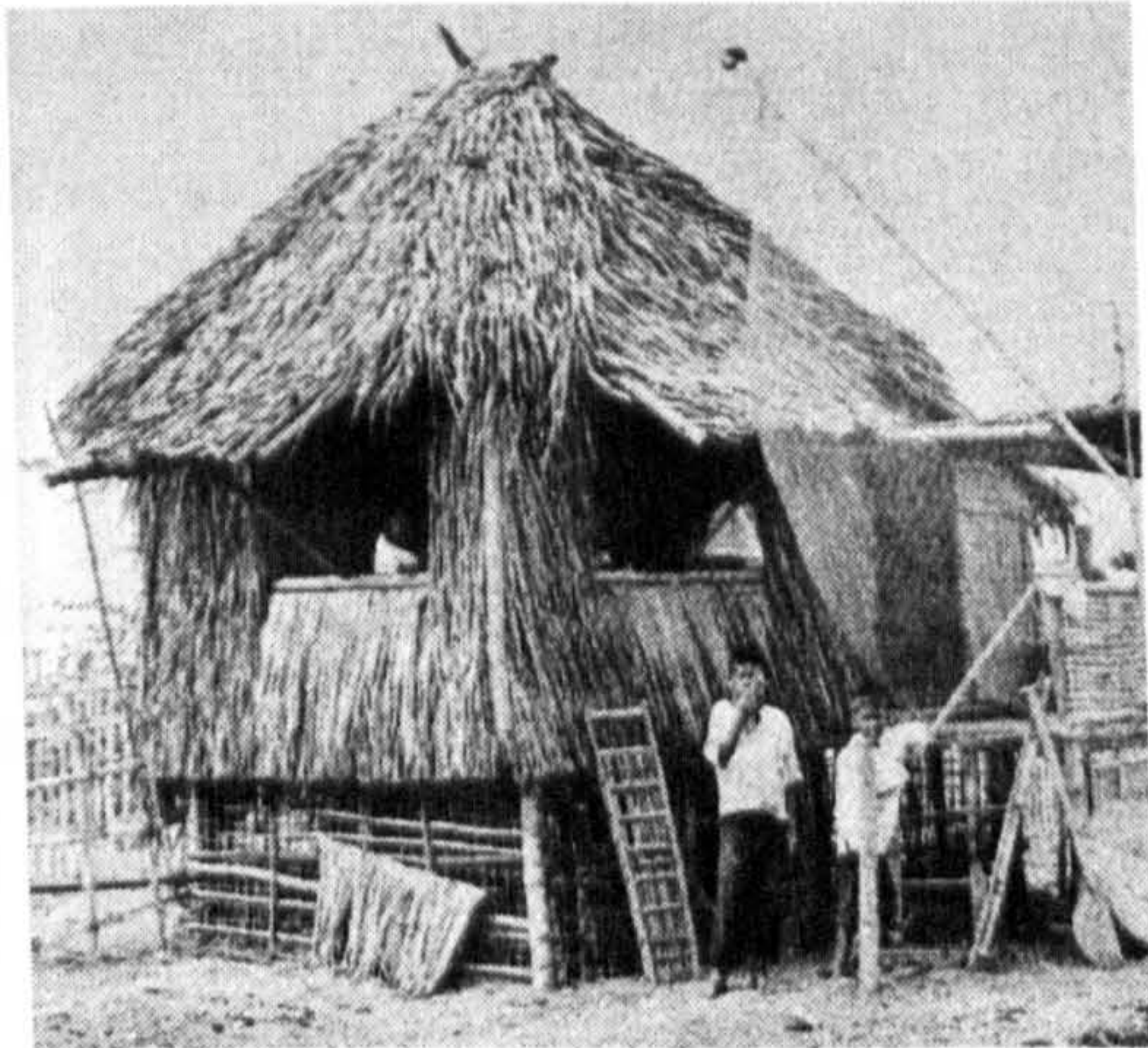
Figure 6.11: Baha-na-kubo . Pre-Spanish houses of the Philippines: elevated from ground with living spaces on the upper floor and storage spaces on the ground floor, post and lintel construction and abundant use of natural materials such as nipa , bamboo and woods. (Sources : Zialcita, 1980:10)
