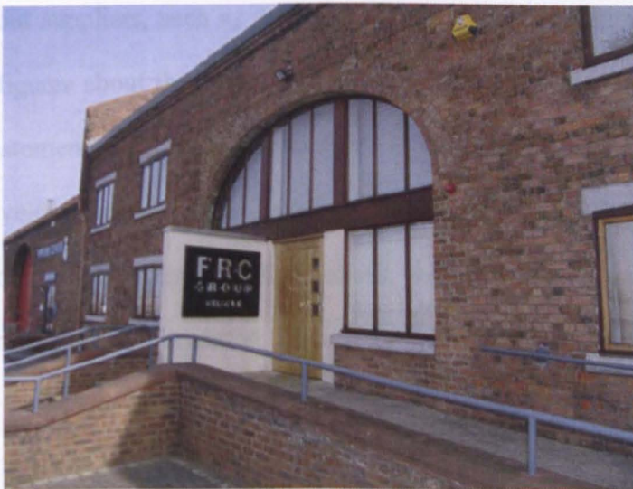
Figure 10.6 The FRC – the new front entrance
