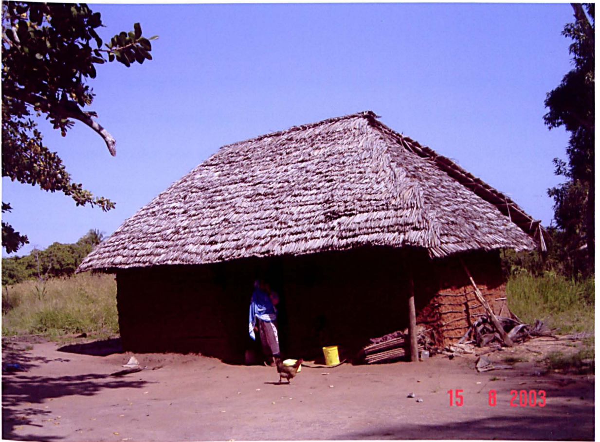
Figure 3.3: A typical house made of mud walls and thatched with coconut leaves.
