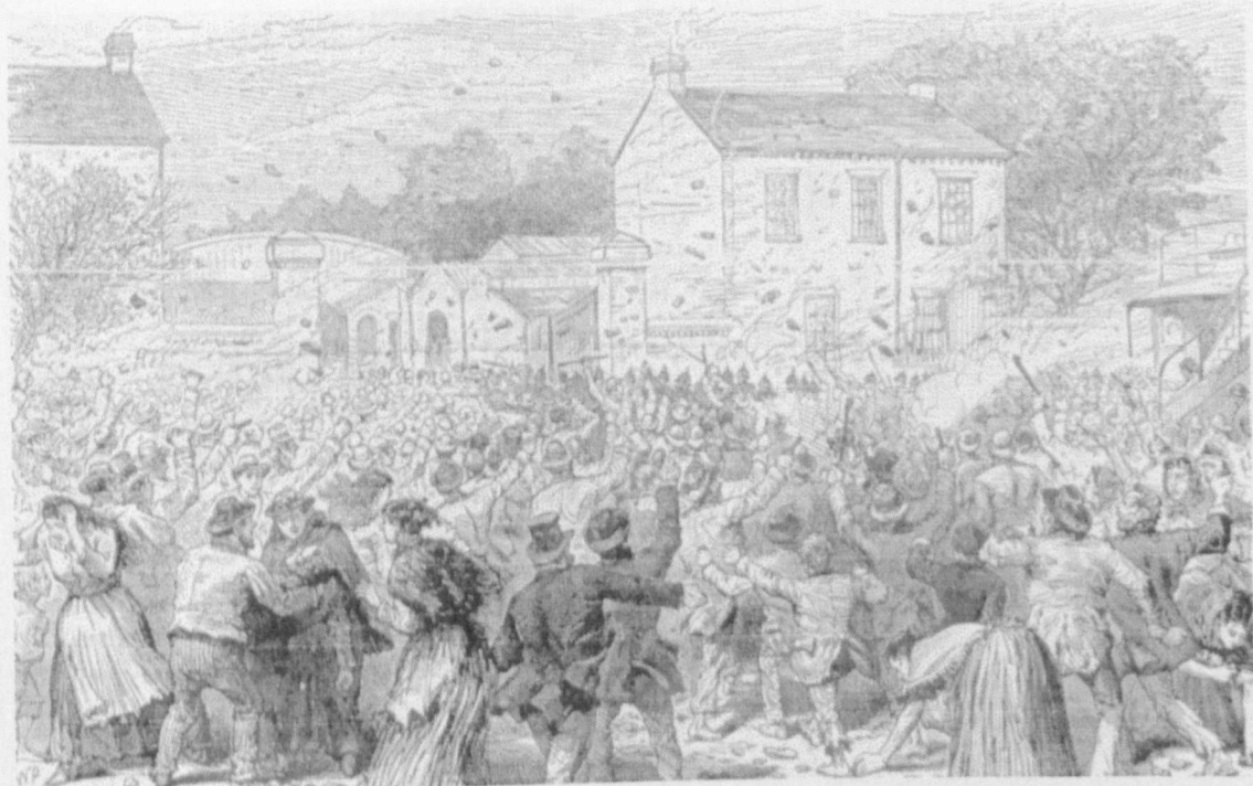
Plate Nine: Mob wrecking the tramway company's depot at Milltown.
