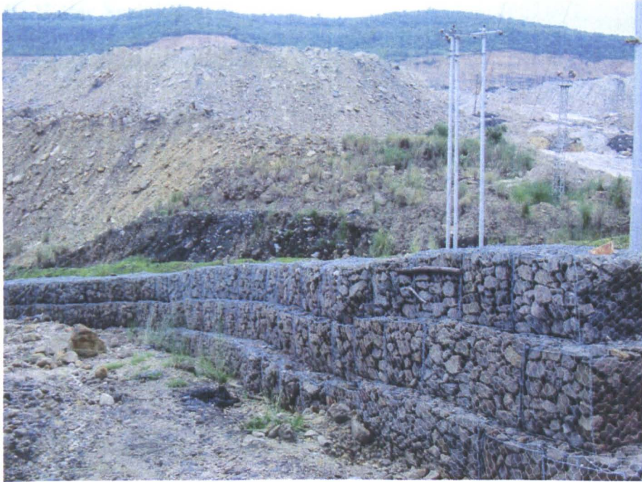
Picture 8. 1. Toe-wall in Kakri OCP (taken by author, 2005)
