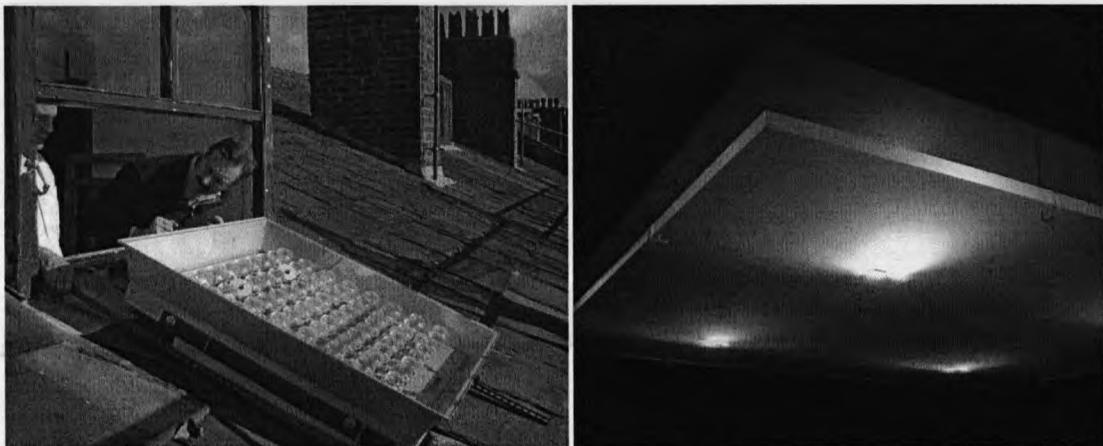
Figure 7.1: Parans solar panel installation in the Uni. of Liverpool (left); Figure 7.2: Parans 'L1-large' luminaire (right).
