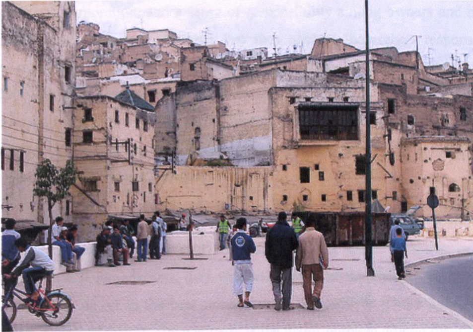
Figure 4-4- Current Condition of the River (Oued Fes), Bukhrareb Area. Photo Taken by the Author in November 2006
