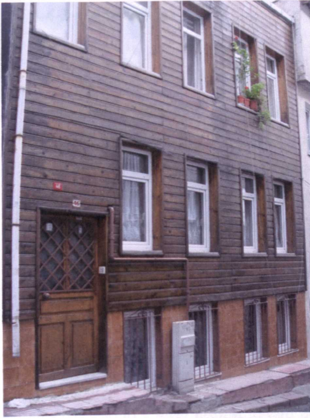
Figure4-21- An Example of a Recently Renovated Timber House in Zeyrek (Picture Taken By the Author, September 2007)
