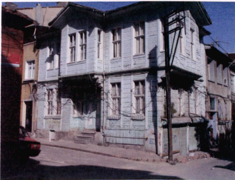
Figure 5-75- This Building Has Benefited From Regular Maintenance by Its Owner and Is Only Resided By One Family (Photo Taken By the Author in September 2007)
