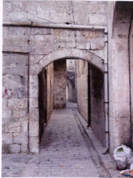
Figure 5-40- A Street in Bab-Qinnisrin Neighbourhood (Picture Taken By the Author in June 2007)
