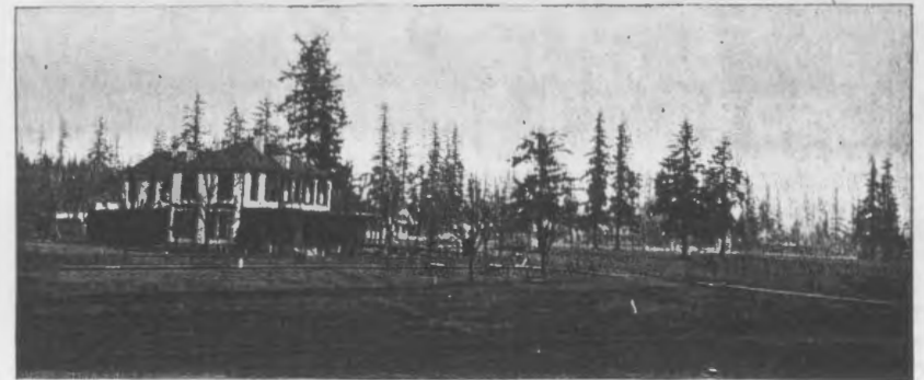
Photographed by the Welster Company, Portland Ore., expressly for THE MIDLAND.
