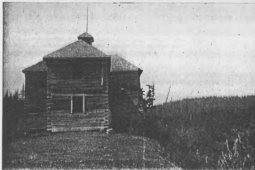
Photographed by the Welster Company, Portland, Ore., expressly for THE MIDLAND.
