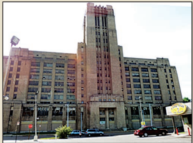
East elevation of Sears Crosstown
