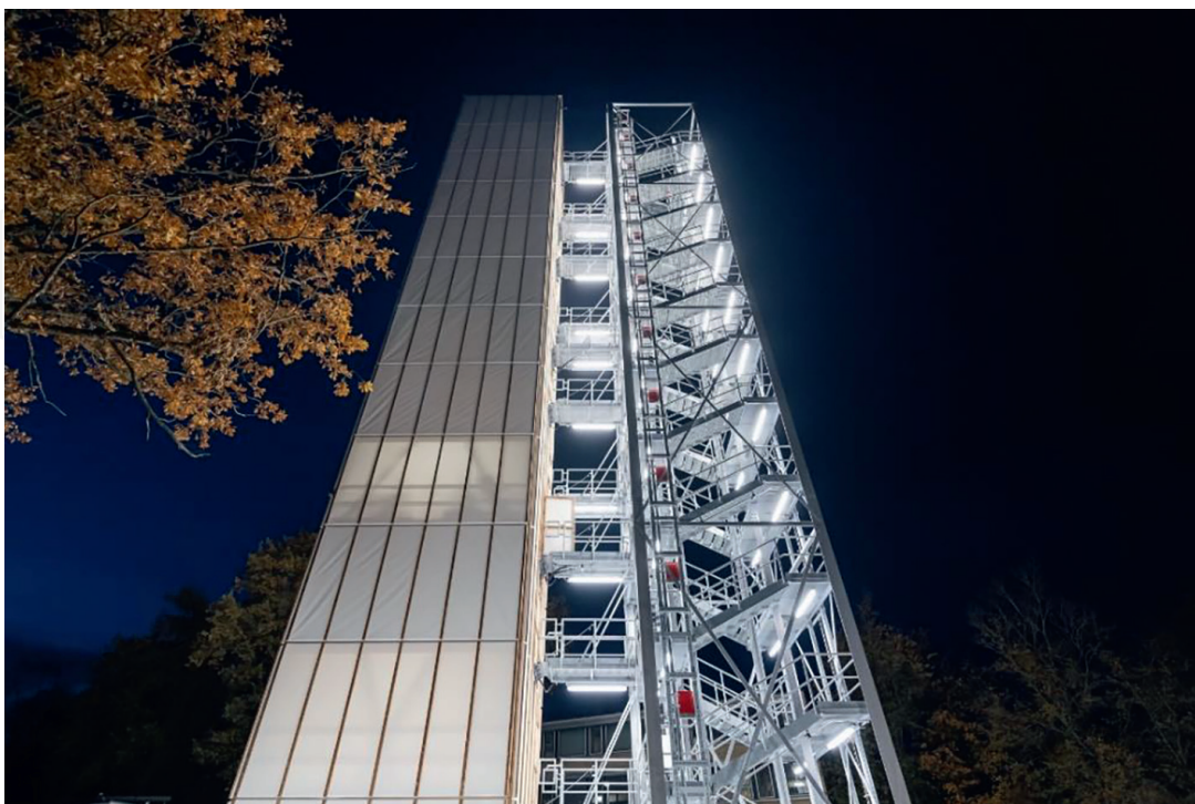
Figure 1. View of the experimental high-rise building D1244, Stuttgart © R. Müller.
