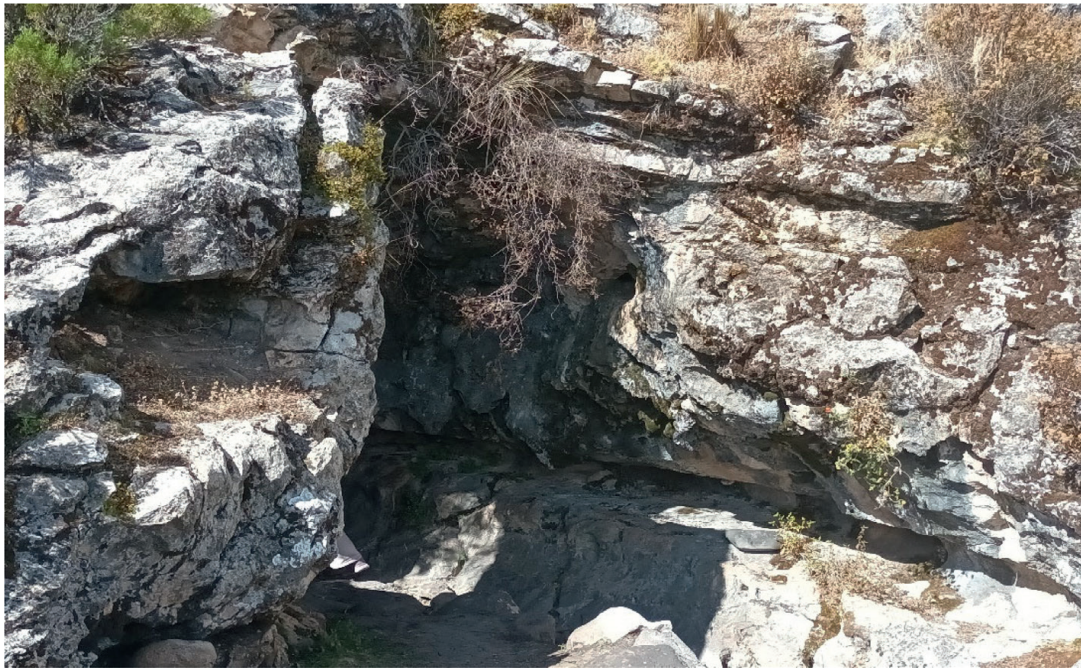
Figure 4. Chinkana Wisccacha. Nota. Close view of the entrance below to the Wisccacha cavern, it has two accesses which are used for the internal walk, from top to bottom and viceversa, with a steep slope between 15° to 25°, located 5 minutes by car from the town of Llamcama.
