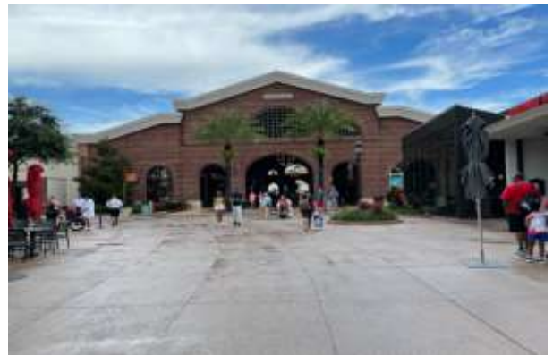
Figure 3. External Plaza, identified as Space #1
