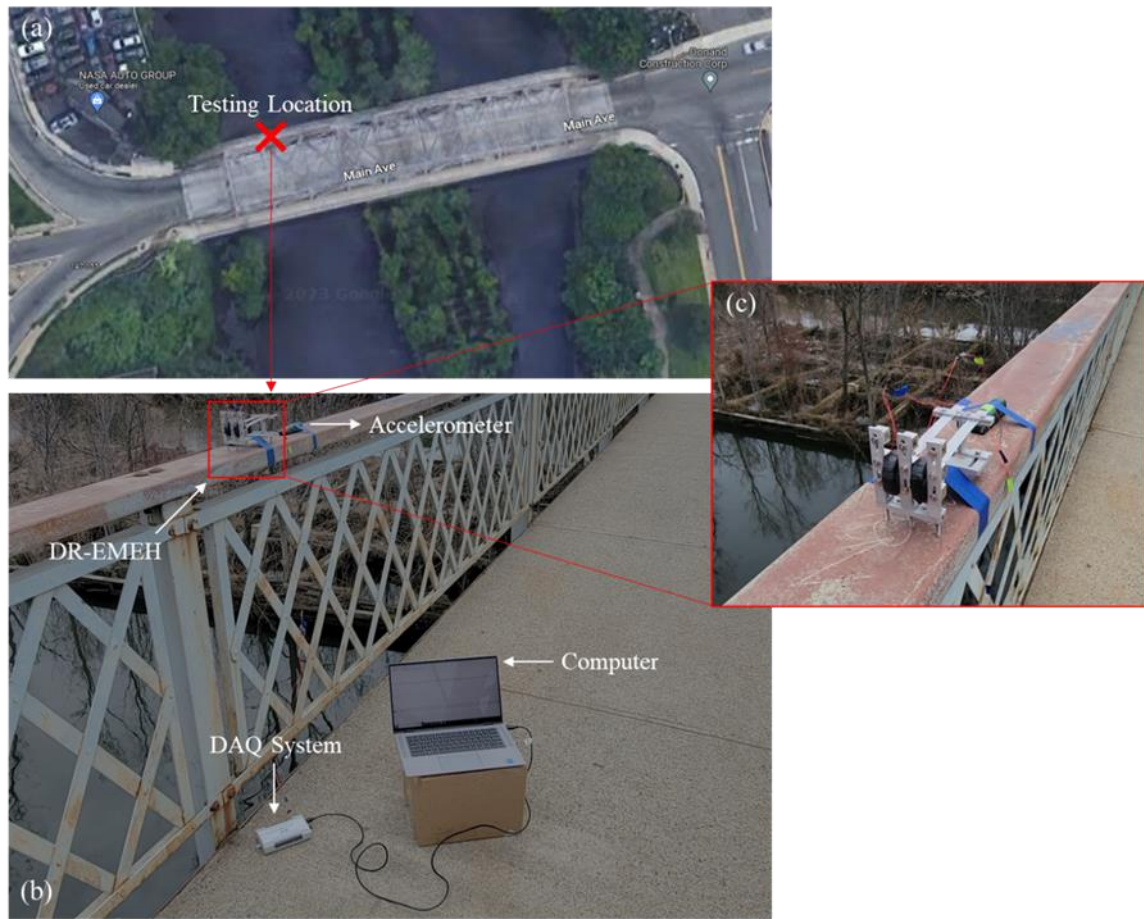
Figure 4.8. Field testing of the DR-EME on the Main Avenue Bridge in NJ: (a) photo of the bridge taken from the Google map with the location of testing marked, (b) testing setup, and (c) mounting of the device on the sidewalk railing.
