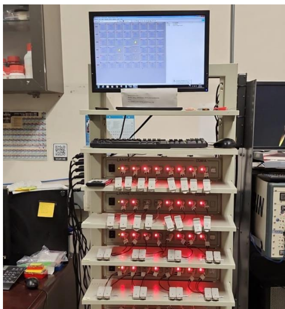
Figure 13: Image of LANHE battery testing system.
