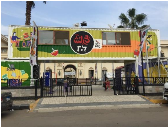
Figure 9. The project has two opposite entrances located on both sides of the project area.
