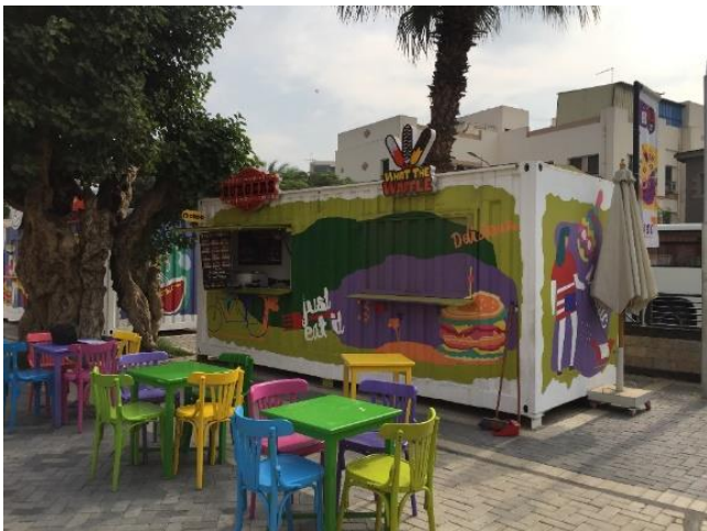
Figure 10. The project uses the Cargotecture concept which depends on reusing the old containers as basic units in the project.
