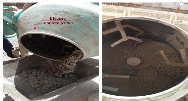
Figure 6 (b). Concrete mixing operation.
