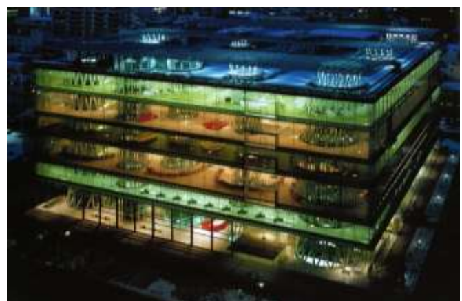
Figure 18. ediatheque building, Senda, japan, 2001 Source: ( https://www.architectmagazine.com/ )
