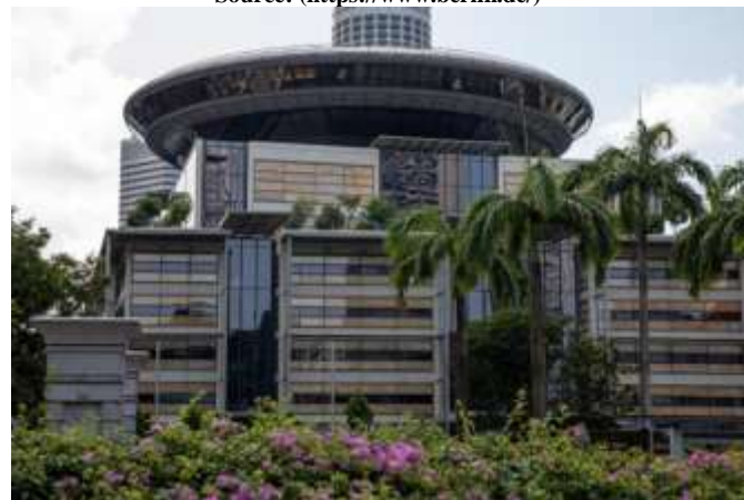
Figure 20. Supreme Court building, Singapore, 2005 Source: ( https://www.fosterandpartners.com/ )
