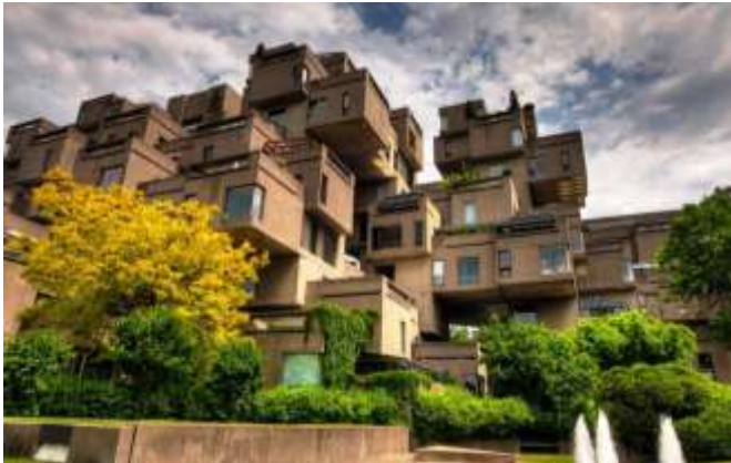
Figure 15. Habitat apartment building, montreal, Canada,1967 Source: ( https://bluprint.onemega.com/brutalism )
