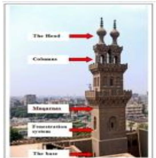
Figure 1: The components of the Minarets: left to right: The Khanqah of Farag Ibn Barquq, The Mosque of Emir Qanibay Qura al-Rammah [author]
