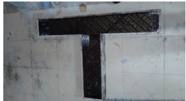
Figure 7. Form works that used for casting
