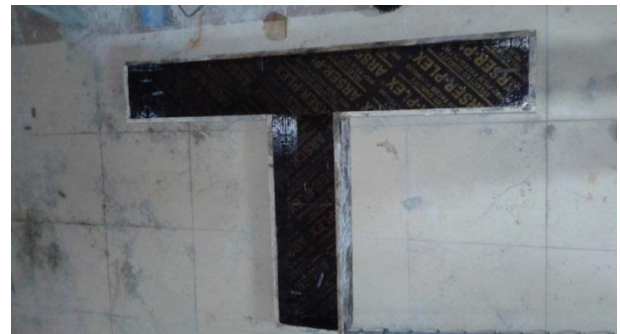
Figure 7. Form works that used for casting
