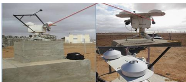
Figure 2. High Precision Meteorological Station installed in the site of Tataouine, Tunisia.
