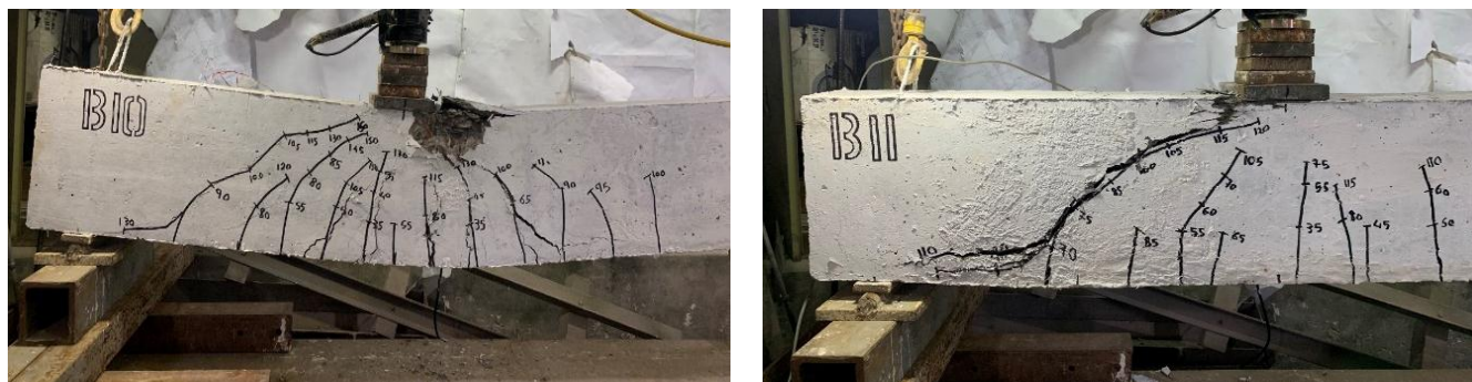
Figure 3. Crack patterns of beams at failure
