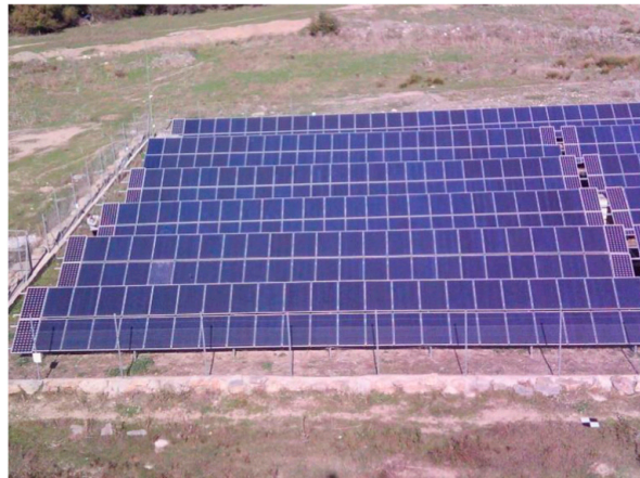
Figure 3. Aerial view of 100 kW PV plant in southern Spain. It can be seen that PV modules with different technologies are located at the ends of the arrays.
