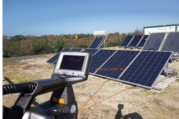
Figure 3. Position of Thermal Camera in front of PV module with \alpha between 0^\circ and 40^\circ .
