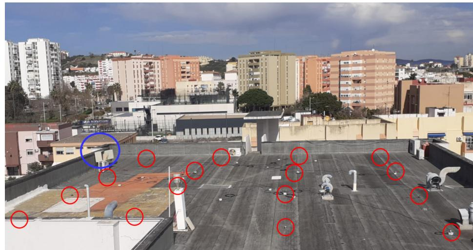
**Figure 11.** WSN deployed at the rooftop of the University building. Red circles indicate pyranometers, and the blue circle locates the position of the router and AC-DC power supply.
