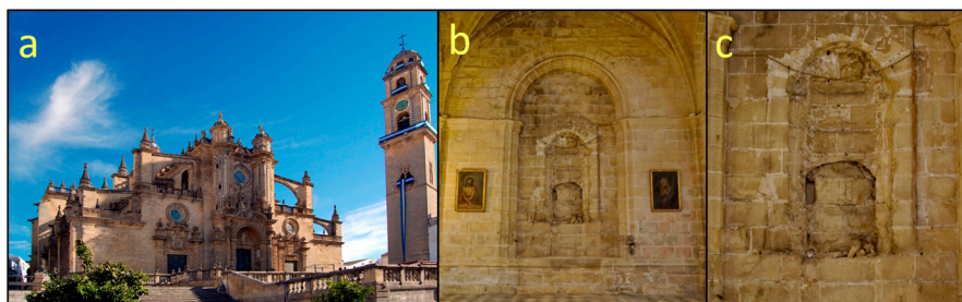
Figure 2. (a) View of the main facade of the Cathedral of Jerez de la Frontera. (b) Stone altarpiece of the Cathedral from which samples were obtained. (c) Detail of the stone altarpiece affected by efflorescence, superficial detachments and sand disaggregation.
