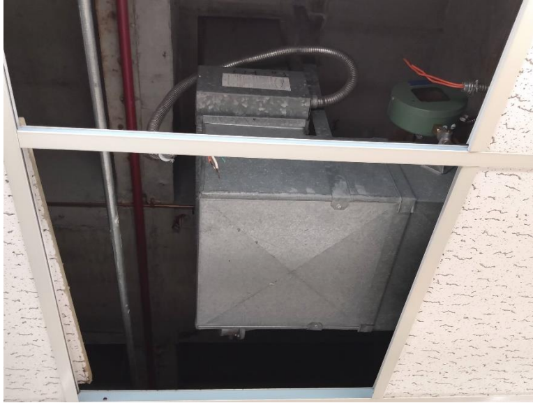
1968-era heating unit in the ceiling of a collections storage area.
