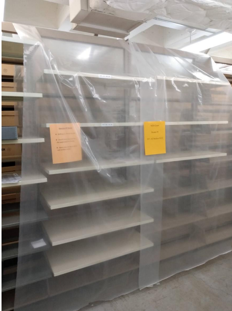
With collections relocated, stacks were draped and heater locations identified with signage.
