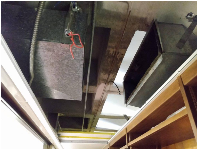
Old heater removed; new one still to be installed.
