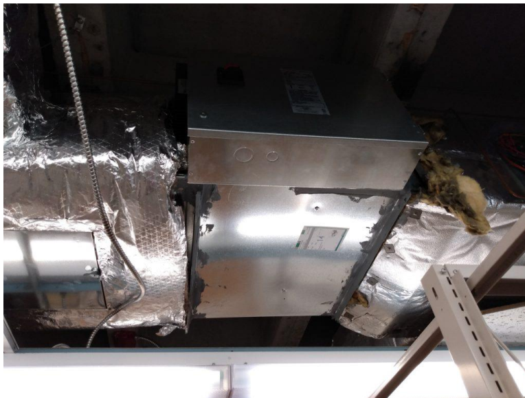
New heater installed in ductwork.
