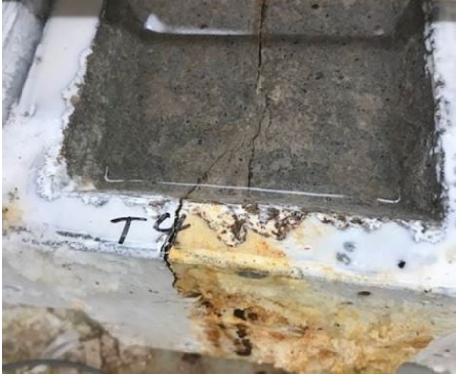
Figure 3.28: Cracking of the concrete in specimen Conv-B-3 during the cracked beam test
