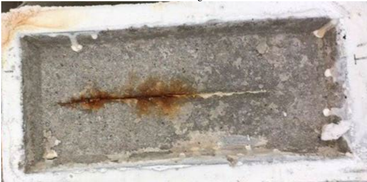
Figure 3.58: Surface staining on the cracked beam specimen with conventional reinforcement
