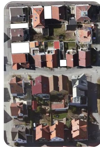
Fig. 71. Open block: In basin 2. Vestre platå there is mostly between open block neighbourhoods. (kart.finn.no)
