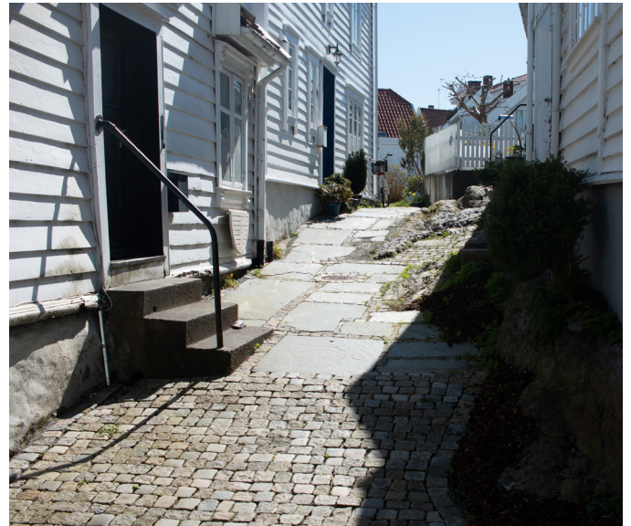
Fig. 53. The paving changes from cobblestone to cut nature slabs in the smug leading to the cherry orchard (IP, 2023).
