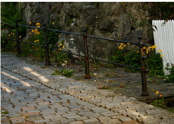
Fig. 55. Horse steps in the cobblestone to help horses with iron shoes walking in the steep streets. An iron railing helps the visitors of today (IP, 2023)
