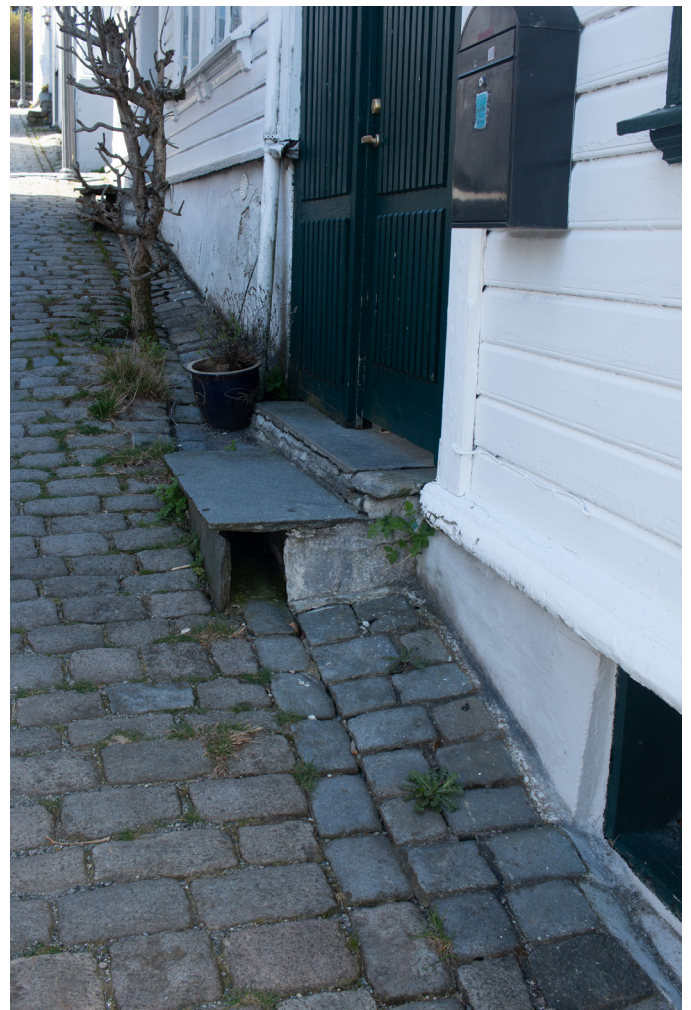
Fig. 54. The cobblestone pavement stops directly in the wall, the closest part is often made with concrete in between the stones, The hole in the stair is to ease the passing of the water so there won't be any built up on the upper side of the stair (IP, 2023).
