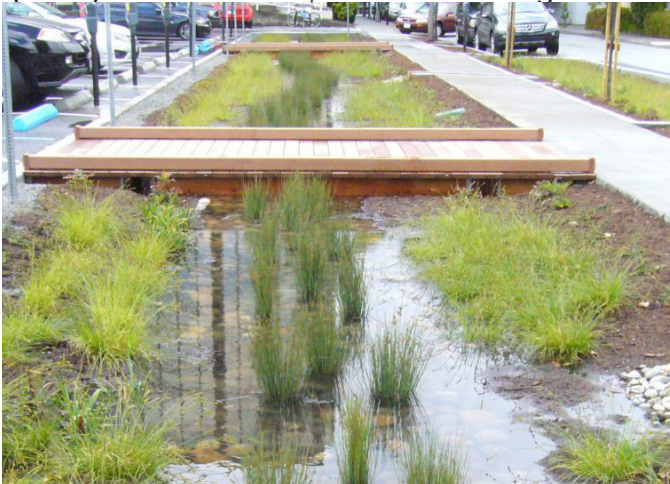
Fig. 17. Infiltration ditch collecting water from nearby parking in San Mateo, USA (Flows to bay, n.d.).
