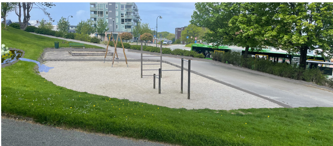
Fig. 81. Illustration of the play area in Rudlå, lowered to be able to collect 129m 3 of water (Picture and manipulation IP, 2023).
