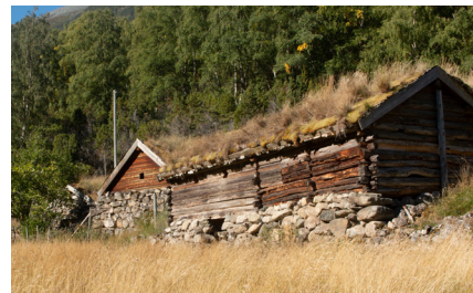
Fig. 14. Traditional Norwegian green roof in Lærdal (IP, 2021).
