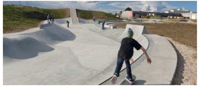
Fig. 21. Skate bowl in Roskilde, it has multiple functions, as a flooding way and retention pool (Åstebøl et al., 2013, Temablad 5).
