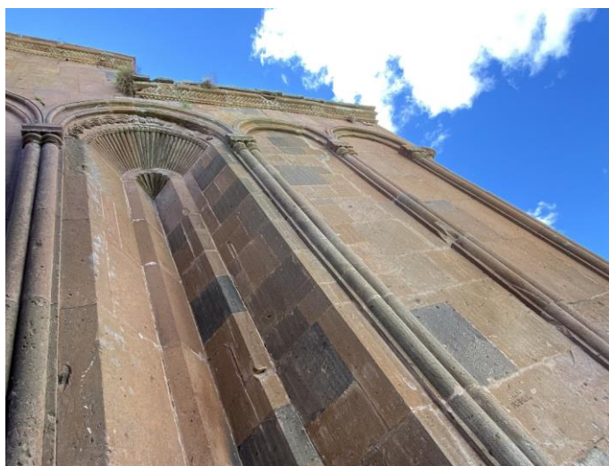
Fig. 7. Part of the northern wall of the Katoghike Church of Marmashen Monastery, Source : own studies.
